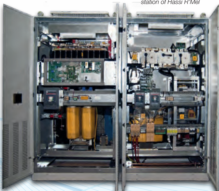
100 KVA inverter installed in the solar power station of Hassi R'Mel
